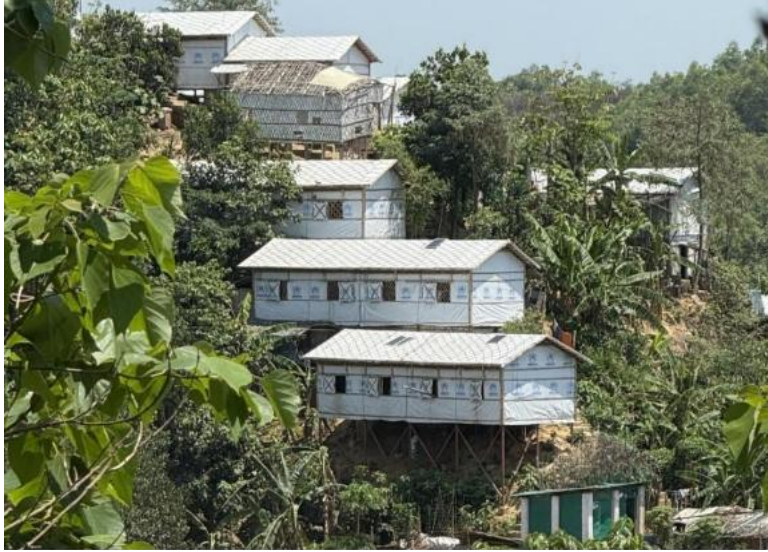
Photo: Shelter Construction in hilly area @ Camp 21
