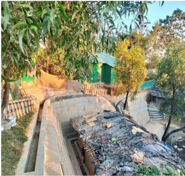
After the intervention: Stabilized slope with improved drainage channels, significantly reducing landslide and flood risks and creating a safer living environment for the surrounding community
