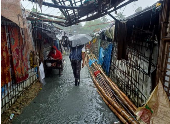
Waterlogging in Block-H, Camp 26 during rain
