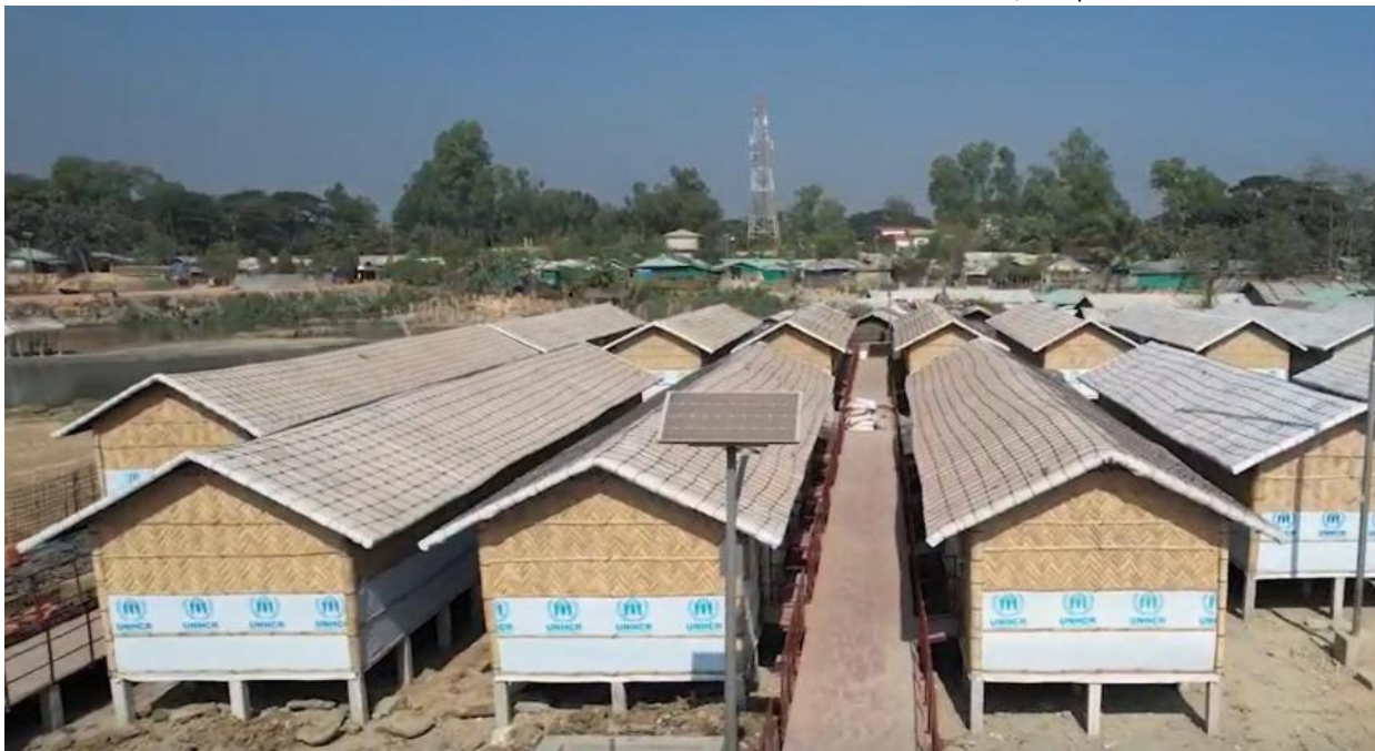
CBS on stilt after construction in Block-H, Camp 26
