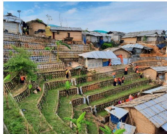
Photo: Slope protection (NBS) in camp 9
