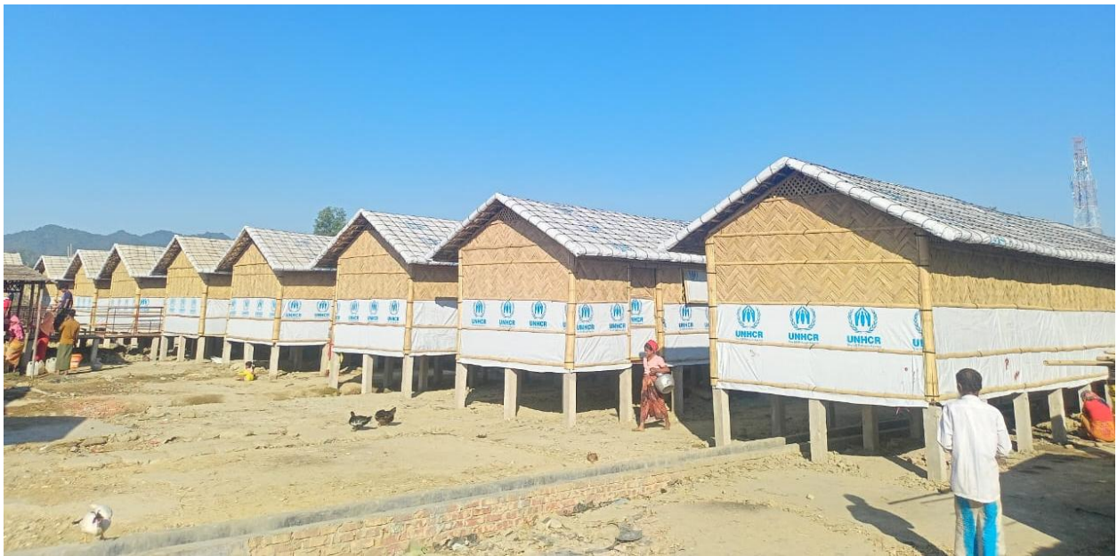
Photo: Stilt shelters constructed in flood-prone areas, Camp 26, Block H
