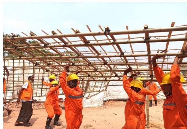
Building Emergency Shelter after the fire incident
