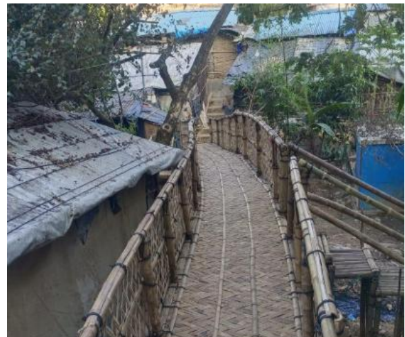
The bamboo bridge ensured the access for the community
