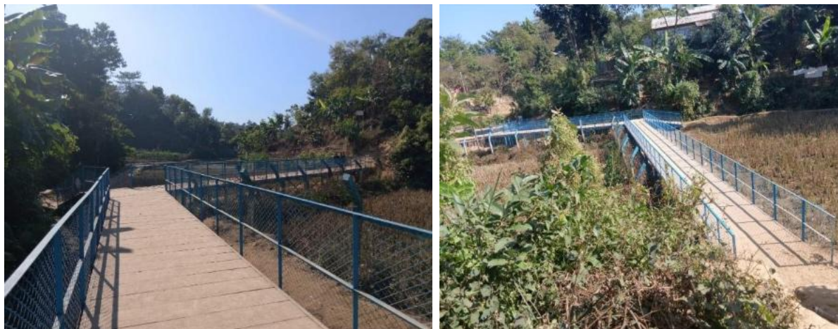
Newly Constructed Four-Face Metal Foot Bridge
