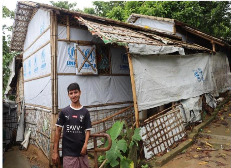
Photo: Emergency shelter Construction
