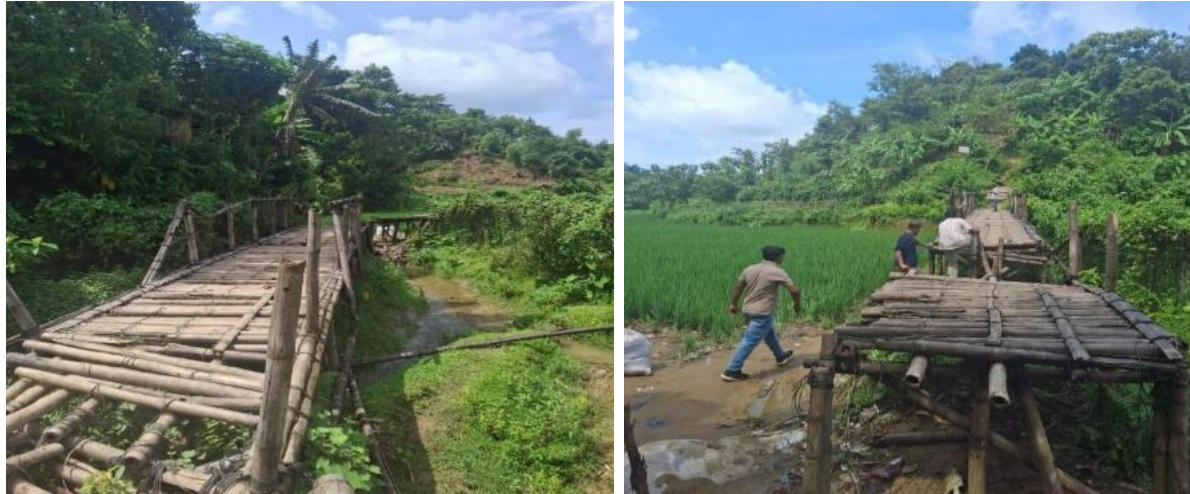
Previous Bamboo Bridge and Context
