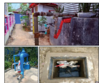
Dedicated Water Outlet with Hose Pipe at Water Network for Fire Response
