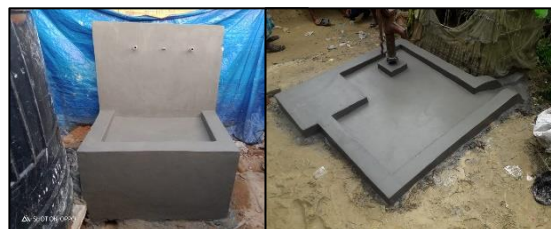
Plastering Work of Hand Pump and Tap Stand Platform
