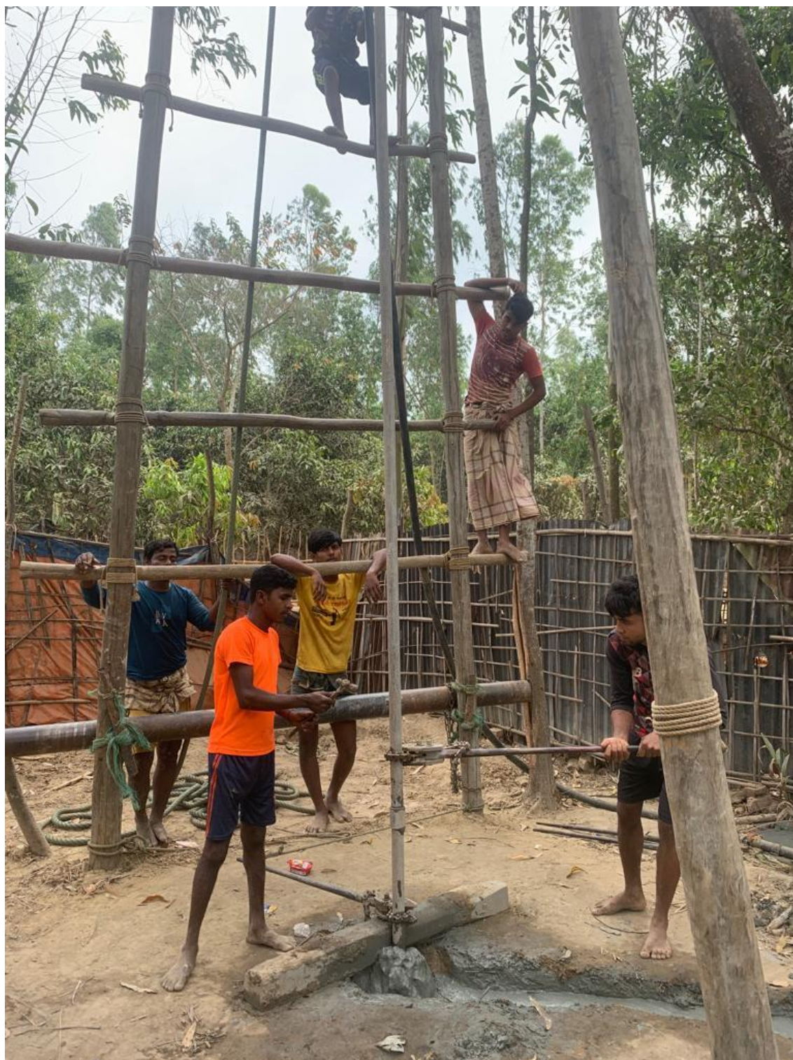
Figure 2.2: Photograph showing drilling technology for the deep monitoring wells
