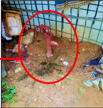
Beneficiary installing own shallow Tubewell inside HH
