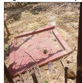
Figure: Hand Pump Head Missing
