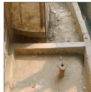
Figure: Non Functional Hand Pump
