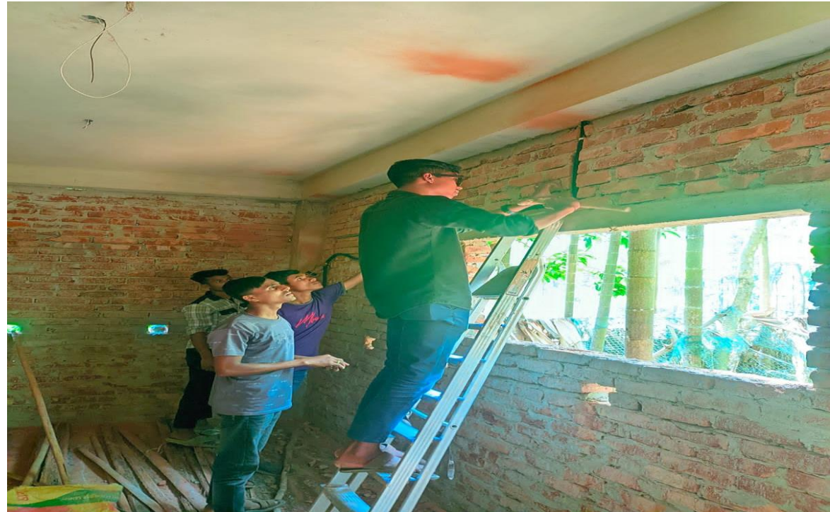
Electrical wiring training @ Plan International
