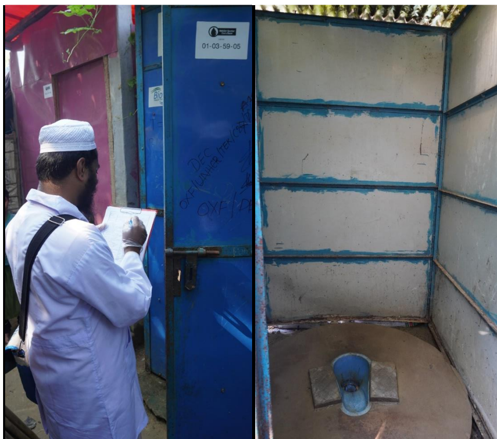
Photograph 2.1: Oxfam constructed 48” dia Biofil toilet at Camp-27, Teknaf Nayapara Camp (ID: Taknaf-Camp 27-SL7-ID-104)
