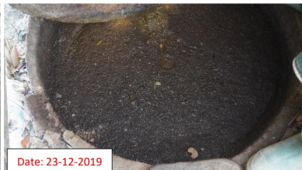
Photograph 2.12: Inside condition of digester of a Biofil toilet at host community near Unchirang Camp-22, Teknaf [ID: Teknaf-Camp 22(Host)-SL1-HH-ID-1120]
