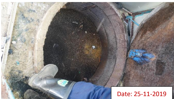
Photograph 2.11: Inside condition of digester of a Biofil toilet at Camp-26, Teknaf Nayapara Camp [ID: Teknaf-Camp 26(C)-SL5-ID-189]
