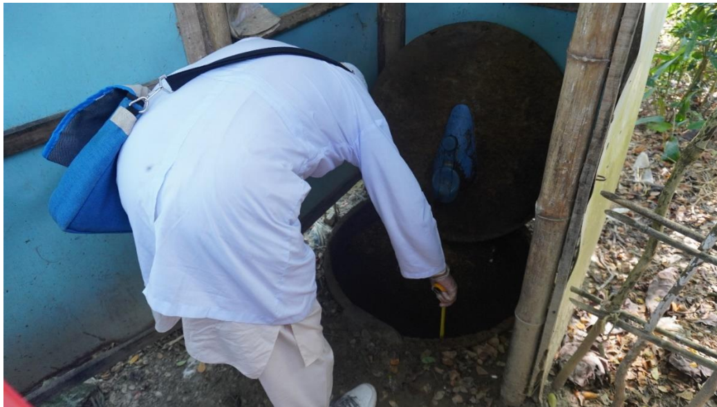
Photograph 2.4: Oxfam constructed 36" dia Biofil toilet at host community adjacent to Camp-22, Teknaf Whykong Camp [ID: Teknaf-Camp22(Host)-SL1-HH-ID-1120]
