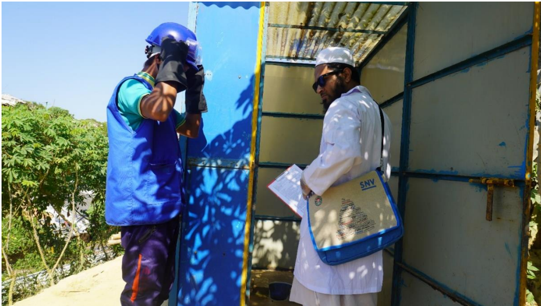
Photograph 2.6: Oxfam constructed Biofil toilet at Camp-12, Ukhia Balukhali Camp [ID: Ukhia-Camp12(B-4)-SL4]
