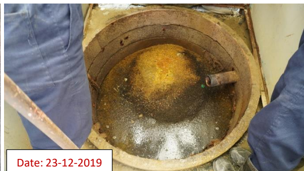
Photograph 2.11: Inside condition of digester of a Biofil toilet at Camp-26, Teknaf Nayapara Camp [ID: Teknaf-Camp 26(C)-SL5-ID-189]
