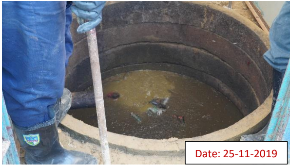
Photograph 2.9: Inside condition of digester of a Biofil toilet at Camp-27, Teknaf Nayapara Camp [ID: Teknaf-Camp 27(B)-SL3-ID-59]
