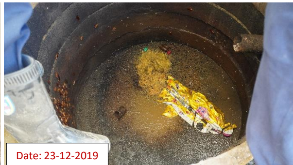
Photograph 2.10: Inside condition of digester of a Biofil toilet at Camp-26, Teknaf Nayapara camp [ID: Teknaf-Camp 26(C)-SL6-ID-147]
