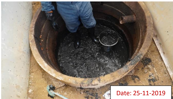
Photograph 2.10: Inside condition of digester of a Biofil toilet at Camp-26, Teknaf Nayapara camp [ID: Teknaf-Camp 26(C)-SL6-ID-147]
