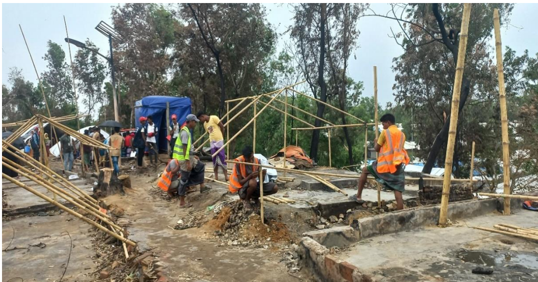
Installation of temporary shelters by volunteers. © Chris Dagnall
