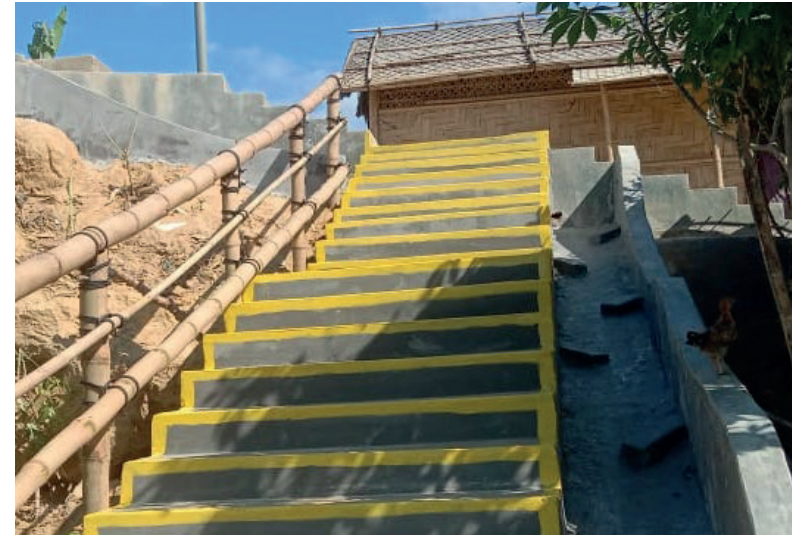
Drainage along stairs – similar to cascade drain in terms of water speed reduction
