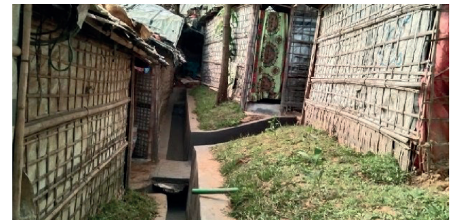
Drain wall height according to the height of surrounding ground and grass covering
