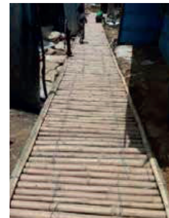
Option: Borak bamboo walkway above drain (N.B. use borak in cross direction) Efficient use of space but increased cost
