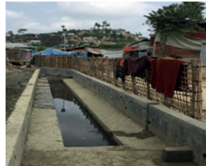
Earthen-base masonry silt trap
