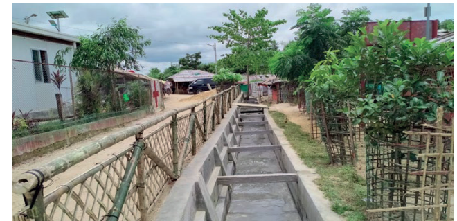
Drain with stepped masonry wall and cross beam
