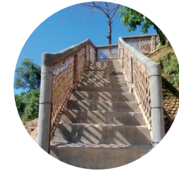
Cement handrail and pole
