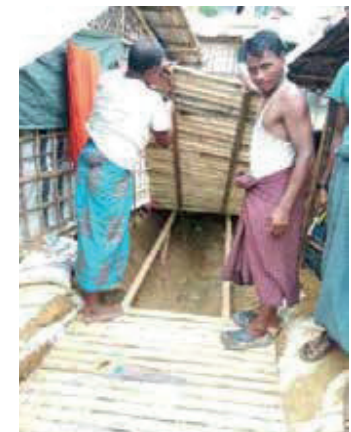
Option: Borak bamboo walkway above drain (N.B. use borak in cross direction) Efficient use of space but increased cost
