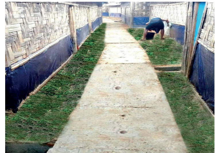
Concrete drain cover
