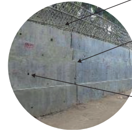
Handrails and fencing along top edge
