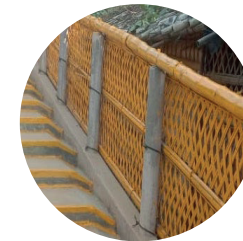
Bamboo handrail and cement pole. The linking between pole and handrail is done through a rebar
