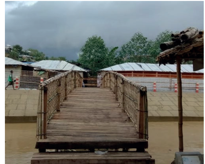
Option: Bamboo bridge with timber deck to reduce maintenance costs!
