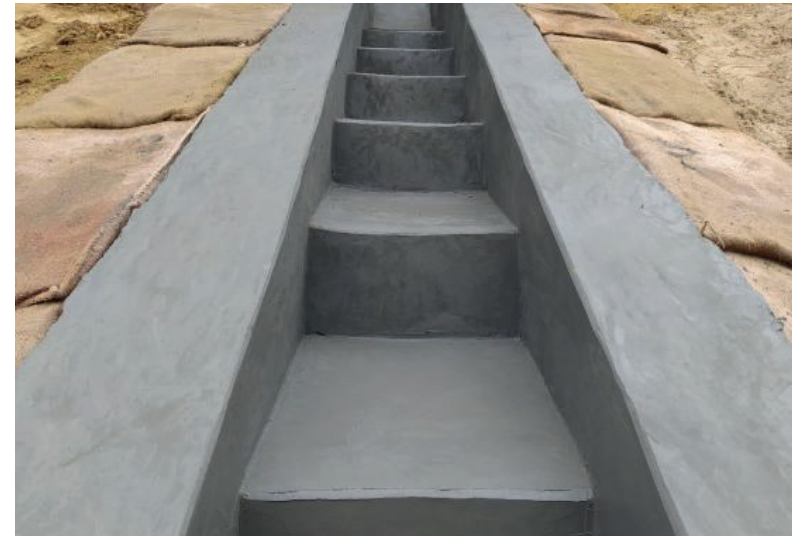
Brick and CC cascade drain
