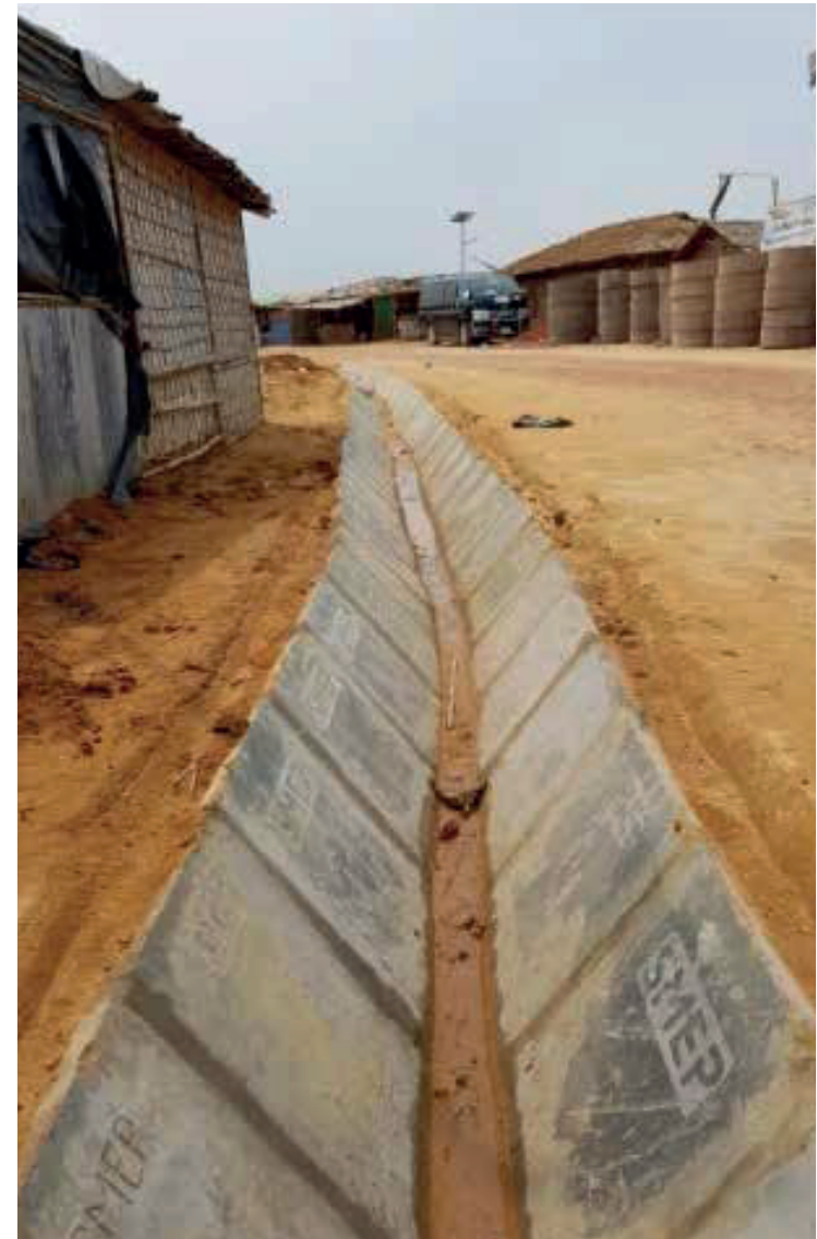
V-drain alongside pathway
