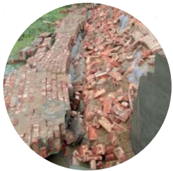
Collapsed retaining wall due to missing weep holes
