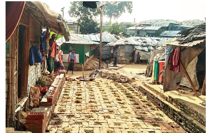
Bricks can also be used to create patterns that promote infiltration.
