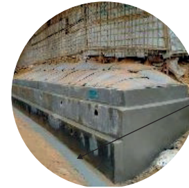
Drain prevents erosion at toe
