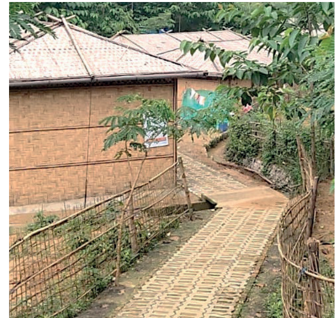
Permeable pavement blocks in camp
