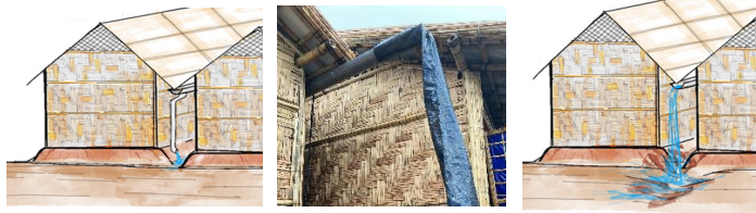
Yes, Gutter all the way to the ground
