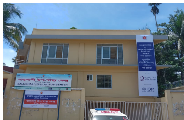
Figure 7: IOM supported renovation of Balukhali sub-center commissioned on 13 July 2023
