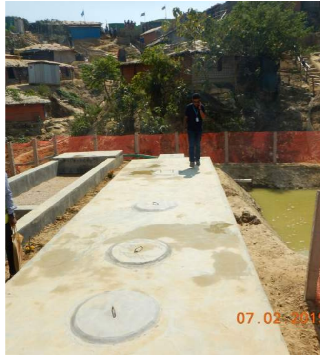
Image 21: Settler and baffled tank
