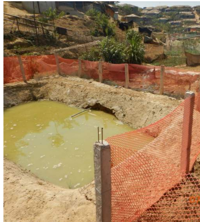
Image 23: ABR polishing pond for liquids
