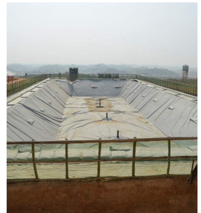
Image 46: Anaerobic Lagoon
