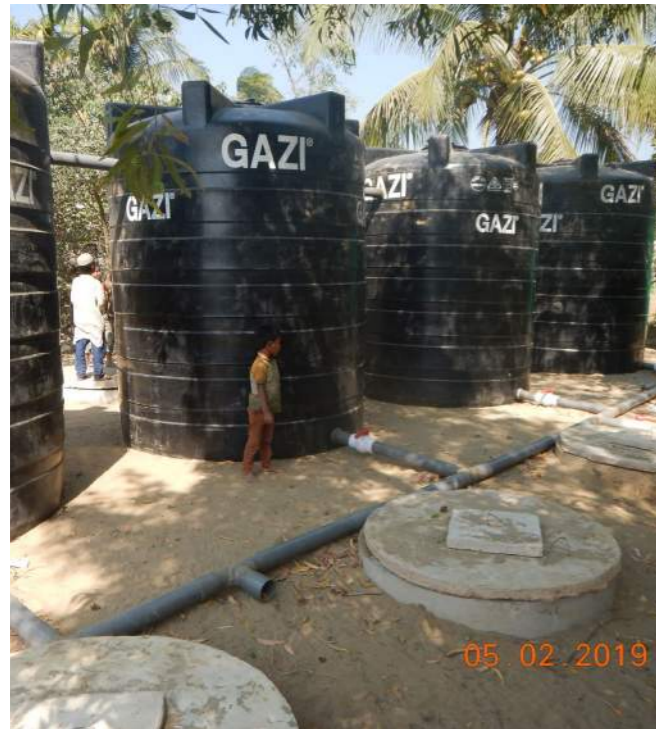
Image 5: NGO 2 - Upflow Filters (under construction)
