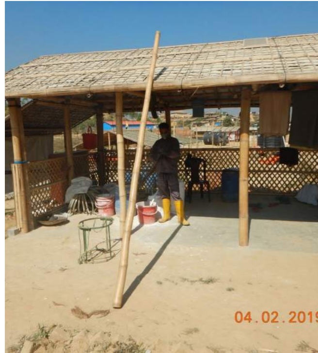
Image 36: Lime 4 - Lime mixing area
