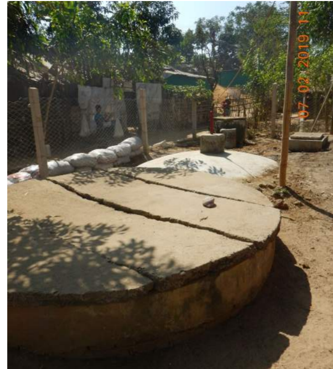
Image 18: Hydraulic Chamber
