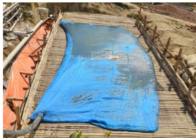
Image 11: GeoTube "bed"
