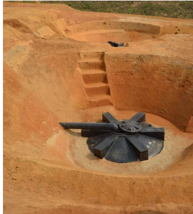
Image 47: Sedimenter with Bristle Filter
