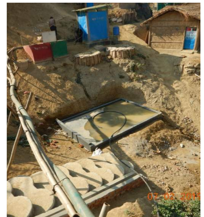
Image 35: Solids storage area (under construction)
