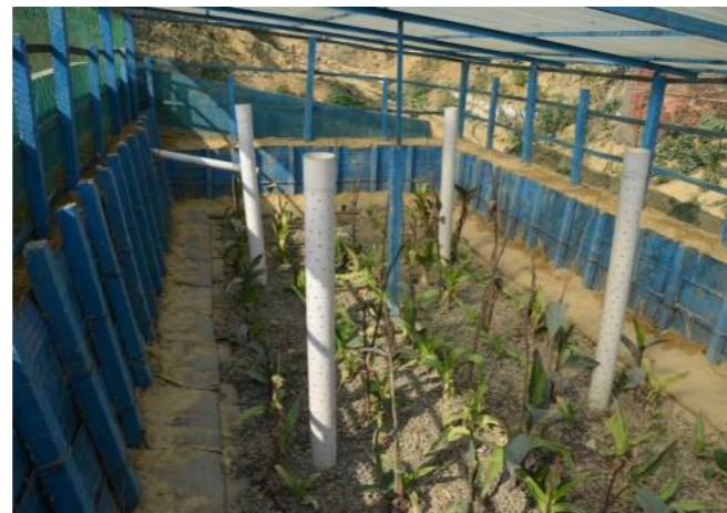
Image 14: Constructed Wetland internal view
