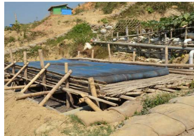
Image 10: GeoTube "bed" with liquid filter below
