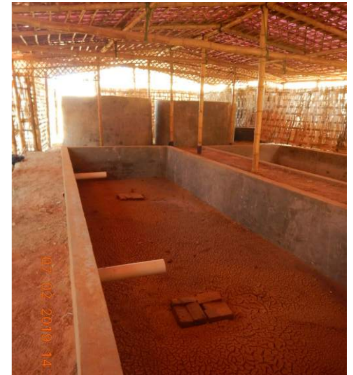
Image 33: Lime 3 - Settlement tank
