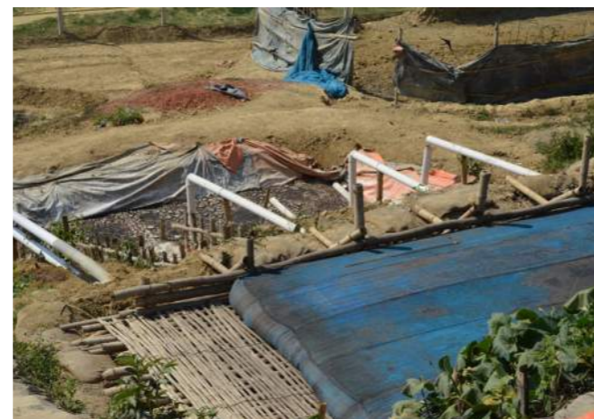
Image 12: GeoTube Liquid Treatment and Solids burial pit in background
