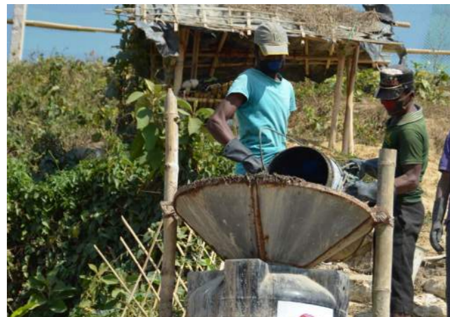
Image 9: GeoTube inlet funnel/screen
