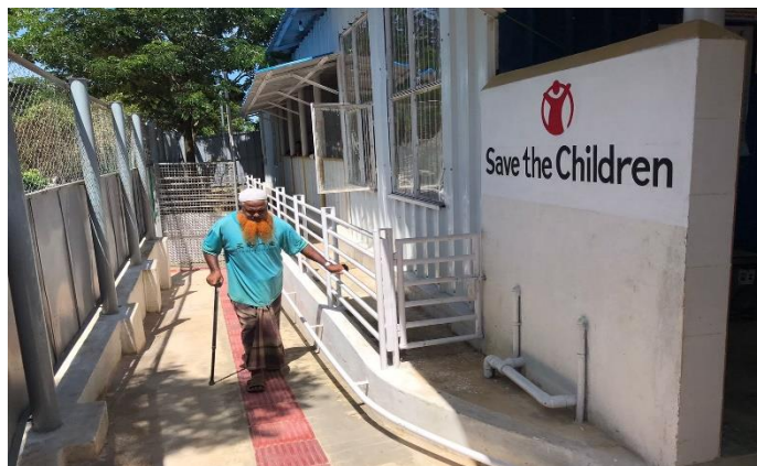
Figure 6: SCI renovated HP with features to improve accessibility
