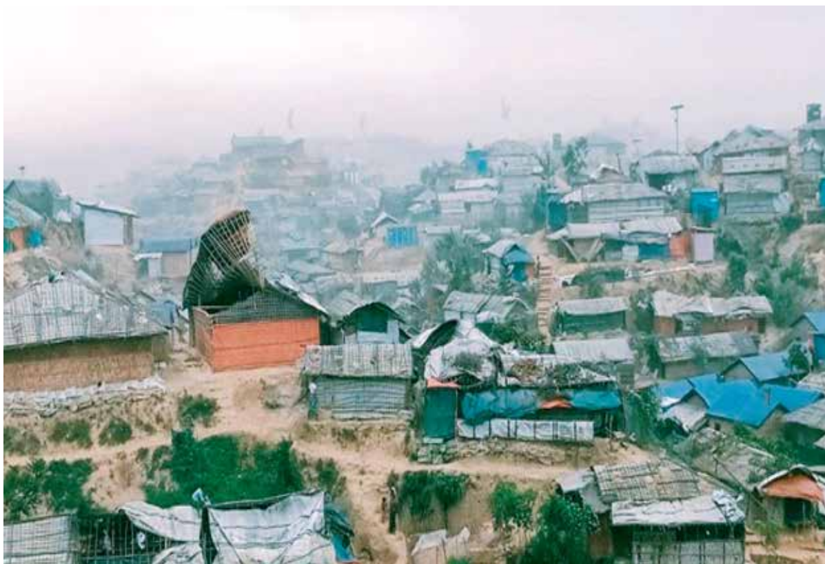
Figure 3: Facilities and shelter damage in camp 18 after short thunderstorm on 25 th February, 2019 (Photo credit: Jony Shahidul Alam, IOM)
