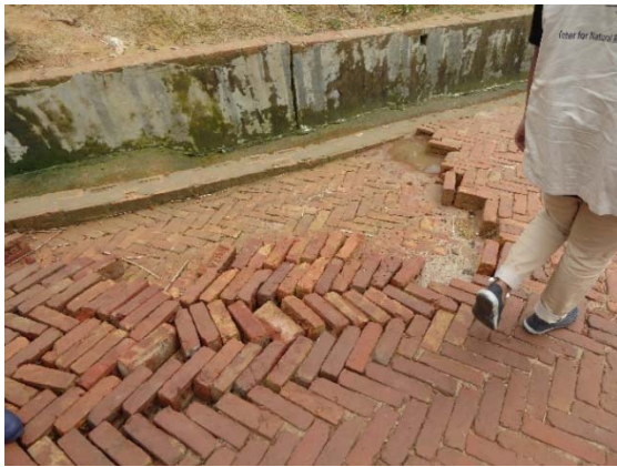
Photo 7.4.19: paved main road
