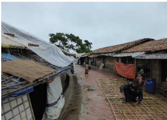
Photo 7.4.3: Workers preparing elements for roof consolidation
