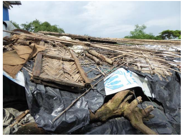
Photo 7.4.14: Typical roof consolidation
