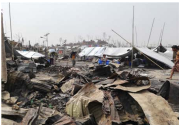
Photo 10.1.1: Debris in the camp 9 on 29 March 2021
