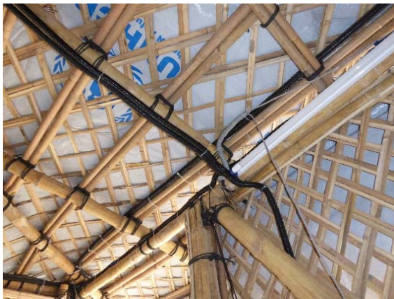
Photo 7.4.1: Registration building just rebuilt, June 2021
