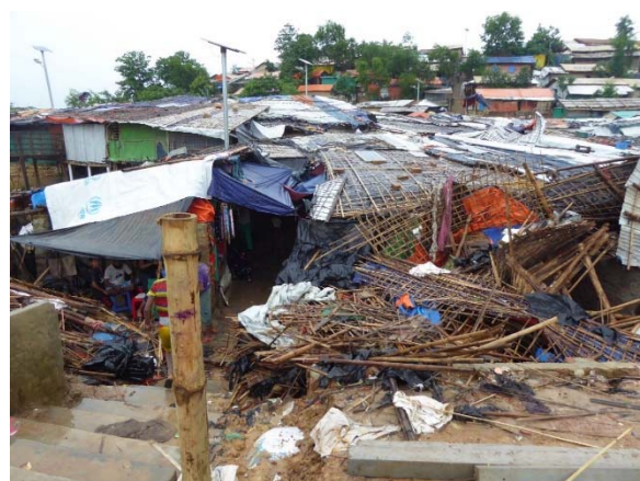
Photo 8.3.2: Market shops collapsed, Camp 4, June 2021
