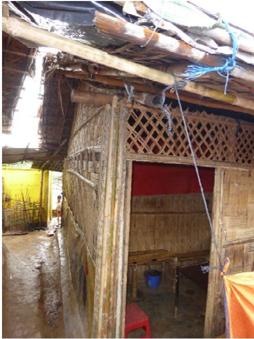
Photo 7.4.5: Inside a shelter
