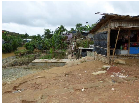
Photo 7.4.20: paved main road
