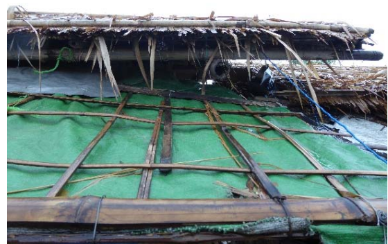
Photo 7.4.4: Typical roof arrangement
