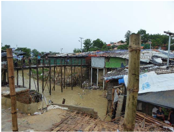
Photo 8.1.3: typical bridge crossing a water stream
