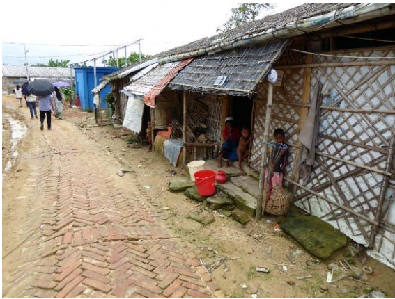
Photo 7.4.13: paved secondary road
