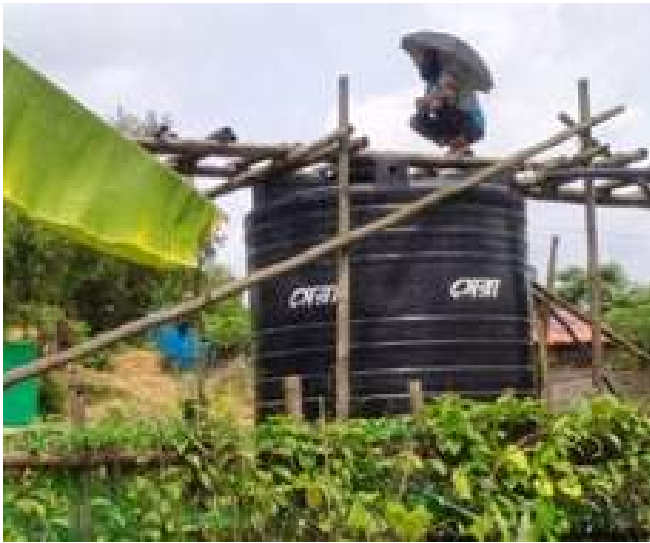
Figure 11: Example of IFSTN transfer tank
