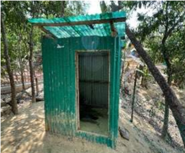
Figure 3: Direct pit single cubicle latrine example
