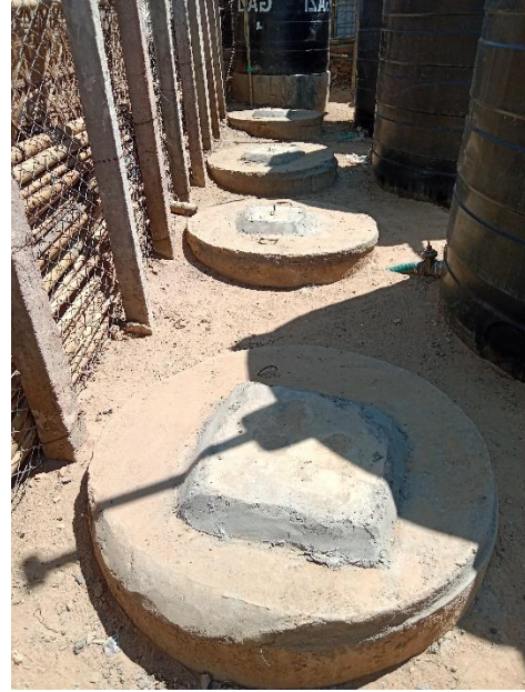
Solids storage pits
