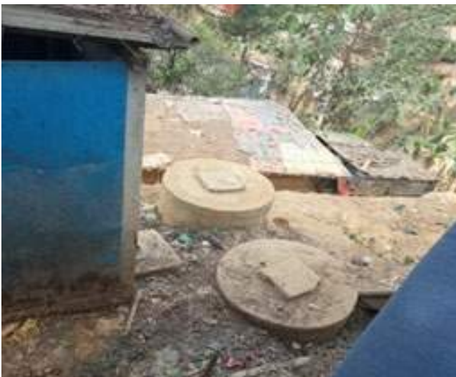
Figure 5: Twin pit offset single cubicle latrine example
