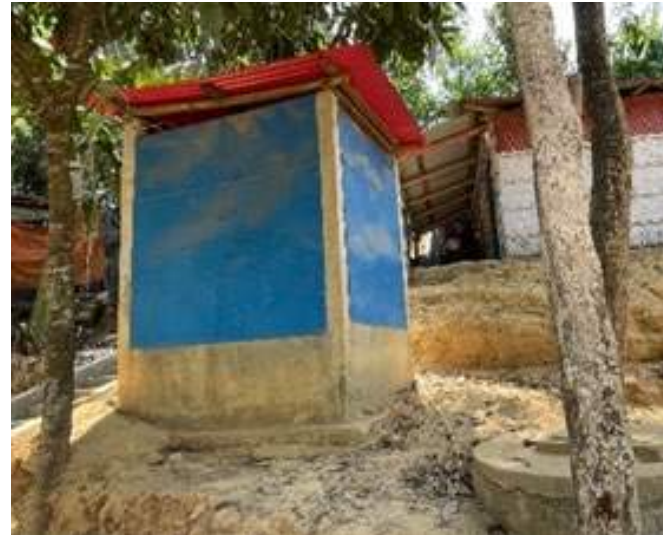
Figure 4: Direct pit with offset soak well single cubicle latrine example
