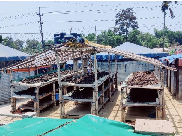
Solids drying and storage
