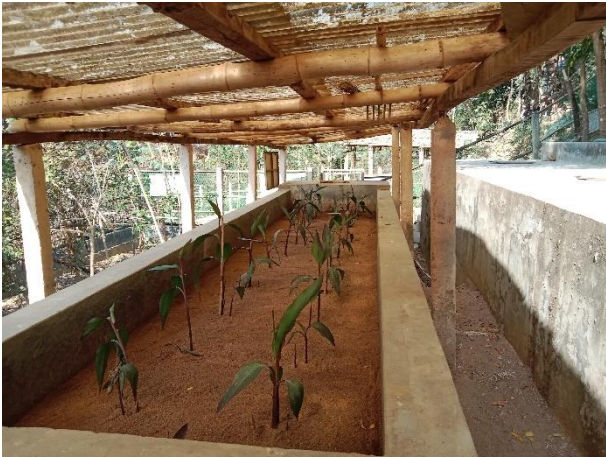
Planted gravel filter
