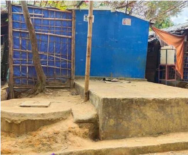
Figure 7: Septic tank with soak pit example
